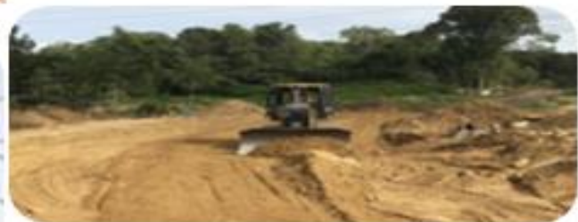
Grading and gravelling of Adawso to Mangoase roads (24.10km)
